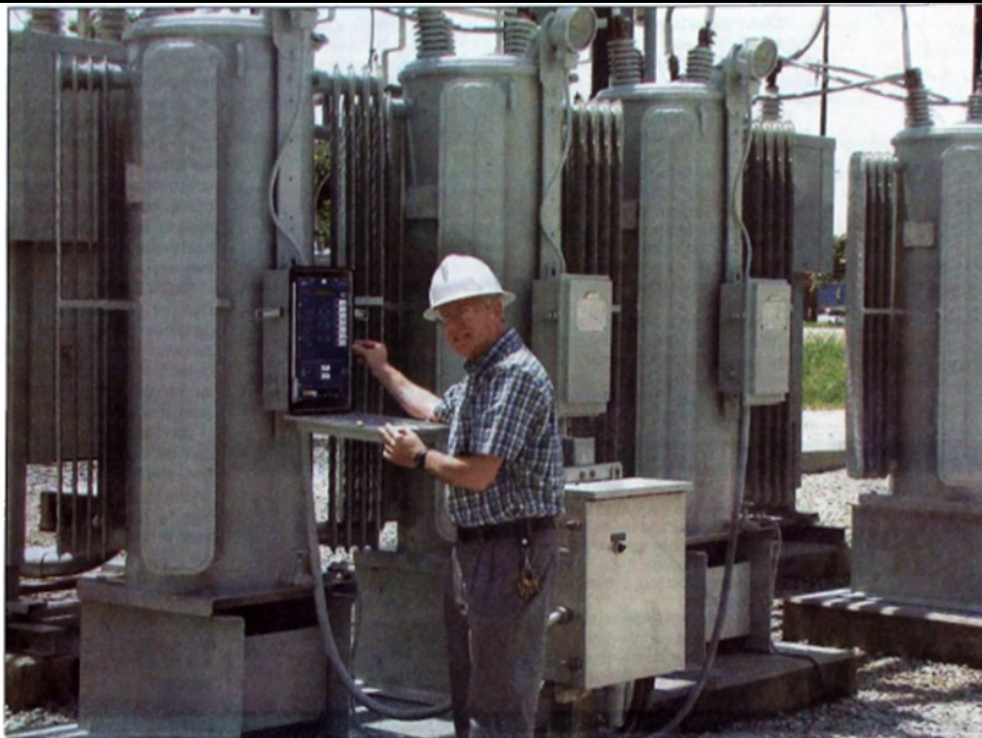
Utilities Director Bill Meecham, here at Covington's largest substation, on Elm Street, is retiring after 20 years with the city. (Staff Photo: Crystal Tatum)
