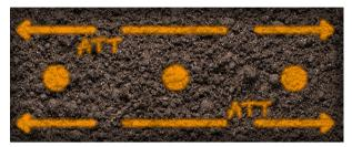
**Duct structures** marked in excess of 36 inches in total will require the underground facility notify the excavator and identify the size of the marked. Any duct structure marked in excess of its actual size will be considered overmarked and will be considered a probable violation of the Marking Standards.
